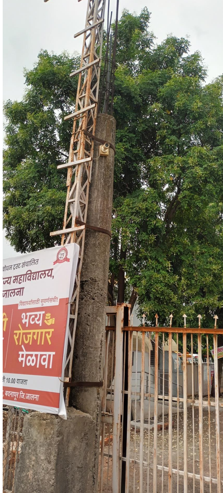
CCTV CAMERA AT ENTRY GATE OF CAMPUS
