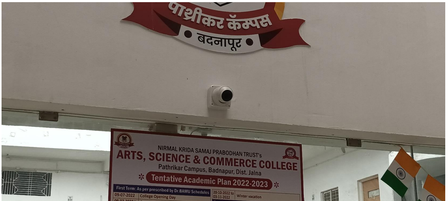
CCTV CAMERA AT ENTRY OF COLLEGE BUILDING
