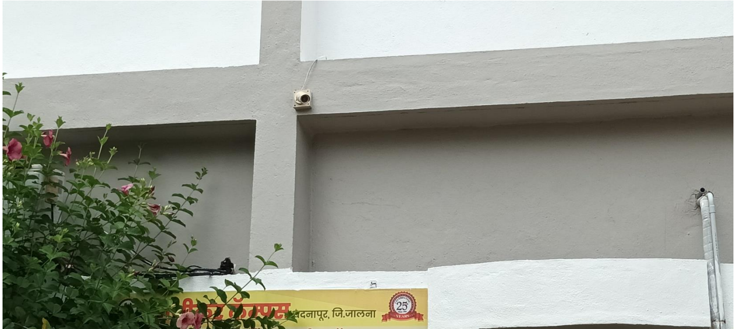
CCTV CAMERA ON COLLEGE BUILDING
